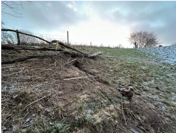
Figure 2.1 Discovered beaver burrow under driftwood after the high-water recede in December 2023 at Waterschap Rivierenland (source Waterschap Rivierenland).
